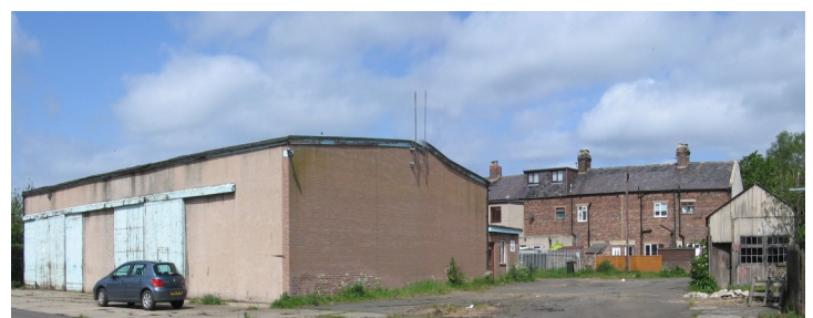
The 1922 old garage and below, the 1960s new garage
