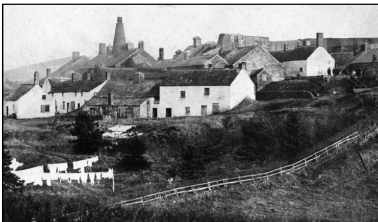
18C Langley Mills where the Greenwich Hospital owners built houses with gardens to encourage workers to stay on site rather than visit a pub on the way home from work
