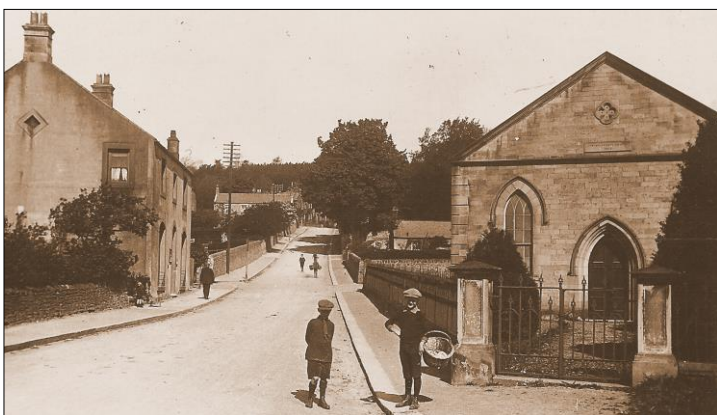
An early post card showing the North Road at Haydon Bridge with the 1863 Congregational Chapel on the right and the Independents' original 1818 place of worship in the foreground on the other side of the road.
