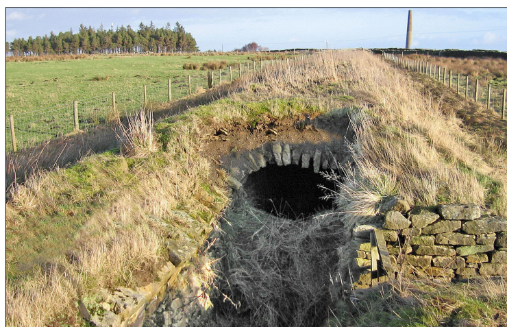
The remarkable horizontal flue, built between 1801 and 1859 from the Langley mills to a flue chimney, can still be seen today.
