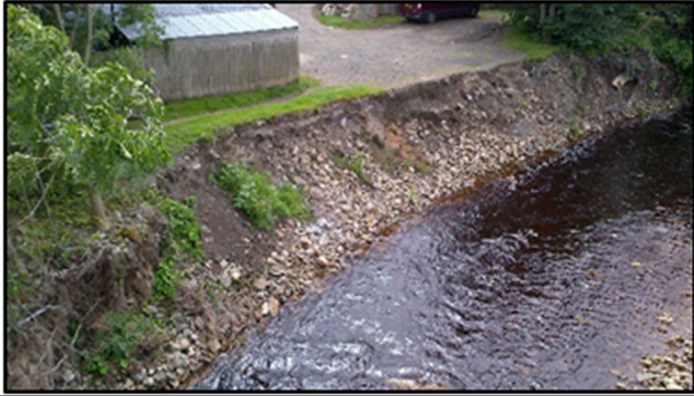
Before – Erosion on the South bank of the River South Tyne, damage caused by the winter 15/16 floods.
