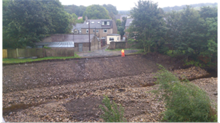
Now – BAM Nuttall are working to repair the bank erosion, using some of the in-channel gravel.
