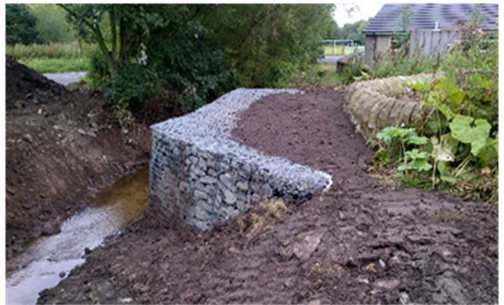
Now – Temple Houses Flood Wall has now been strengthened by gabions.
