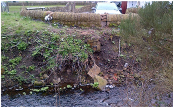
Before – Temple Houses flood wall and the damage underneath caused by the winter 15/16 floods.
