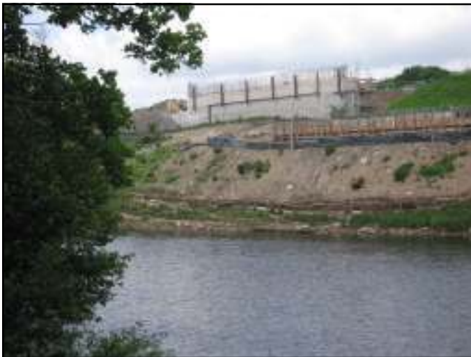
May 2008 views of the north abutment and the east river pier under construction for the South Tyne Viaduct of the Haydon Bridge Bypass
