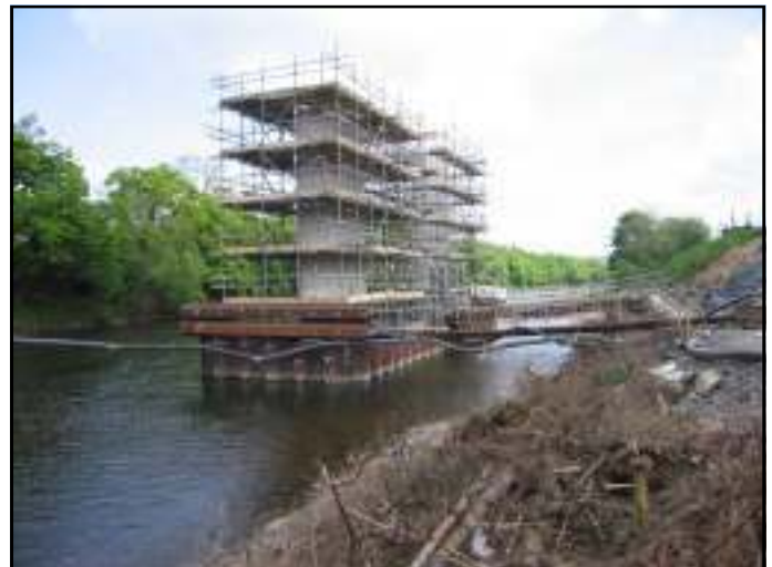
May 2008 views of the north abutment and the east river pier under construction for the South Tyne Viaduct of the Haydon Bridge Bypass
