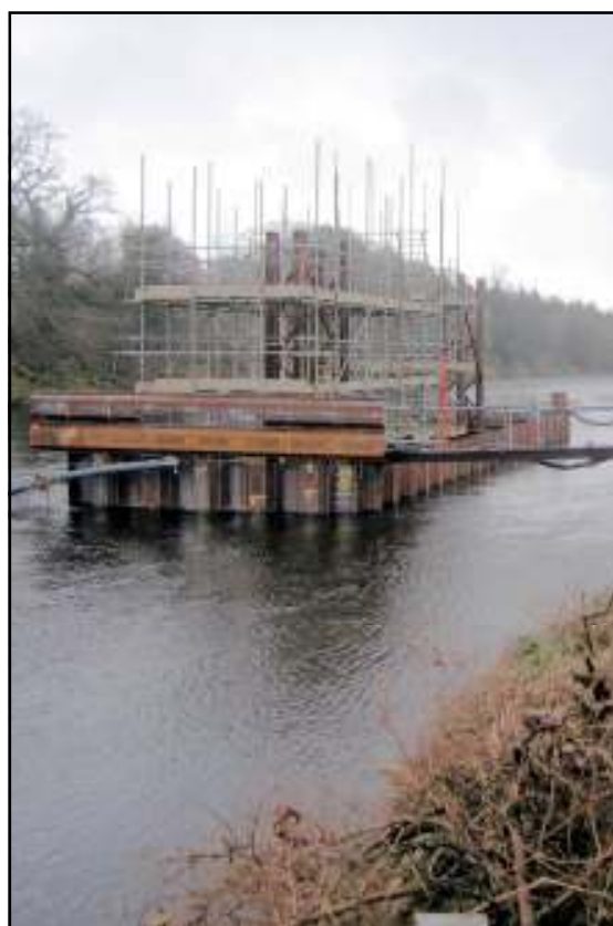
WORK ABOVE GROUND ON THE PIERS OF THE BRIDGES IN GEE'S WOOD AND THE RIVER TYNE FOR THE SUBSTRUCTURE OF THE HAYDON BRIDGE BYPASS (see page 9)
