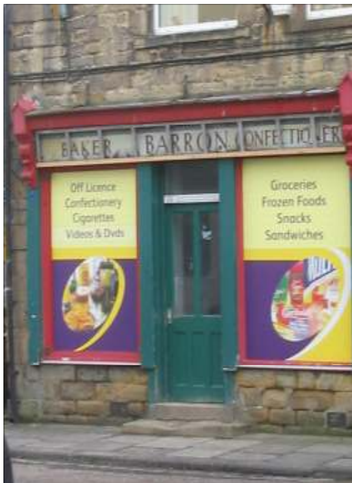
Barron's shop sign revealed during work to convert the Premier Express shop to accommodation. February 2007.
