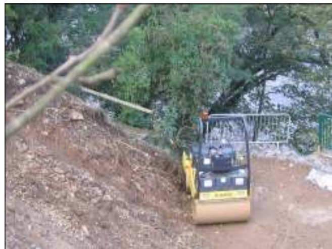
Looking down from the old road onto the new platform.
