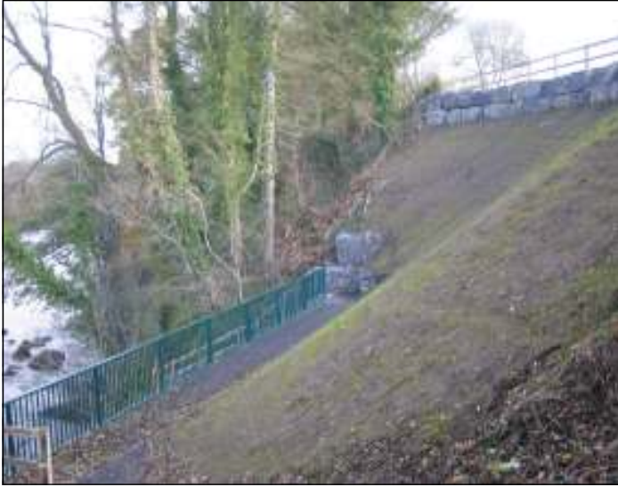
The path to the Spa Well looking east from the old path towards the new platform (belvedere) . The old road is beyond the railings top right.
